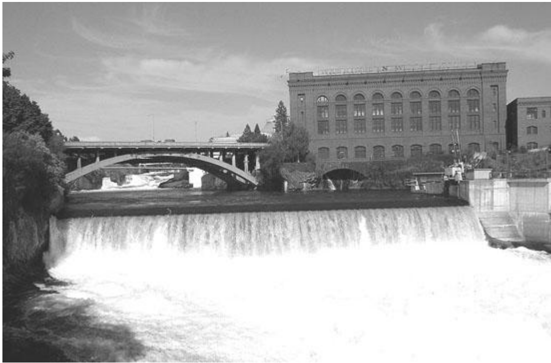
The Monroe Street Dam on the Spokane River.
