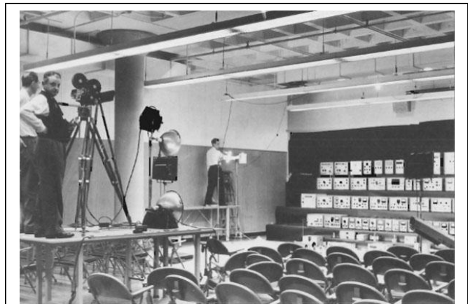
Imagine the troubles of assembling all these 350 instruments and waveguide items into the auditorium of Bldg 5. This Measure Magazine picture shows the setup.
