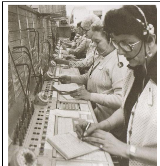
Corporate telephone system to retire (PBX/Lobby 1U, circa 1977)
