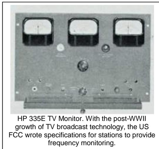
HP 335E TV Monitor. With the post-WWII growth of TV broadcast technology, the US FCC wrote specifications for stations to provide frequency monitoring.
